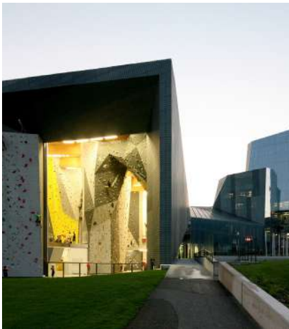
Salewa Headquarters, Bolzano/Italy (2007-2011)
