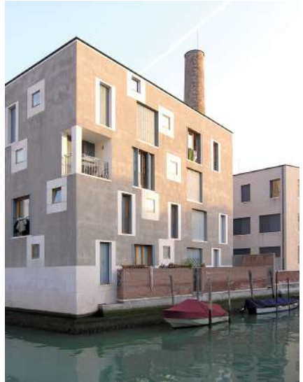
D Residential Building, Venezia/Italy (1997-2003)
